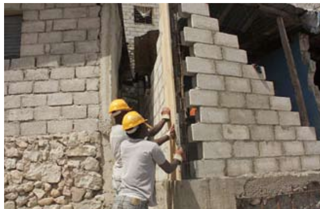
Retrofitting works at Villa Rosa
