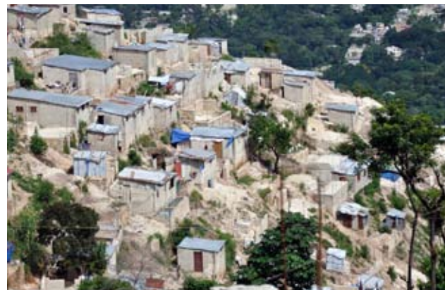
Self reconstruction: new development above Jalousie
