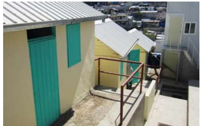
T-shelters constructed at Ravine Pintade
