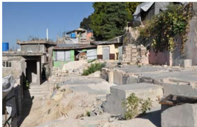
Morne Hercule, housing rehabilitation and reconstruction area
